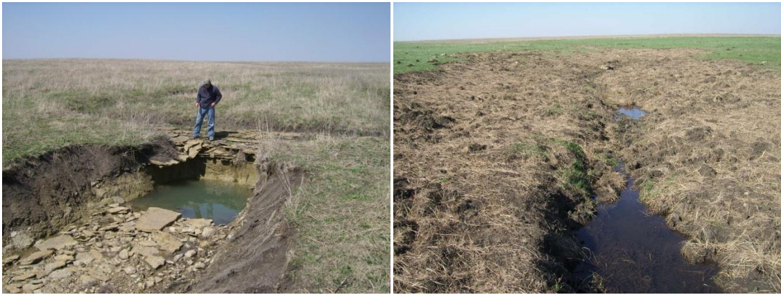
Dry Creek North Headcut, before (left) and after restoration construction.
