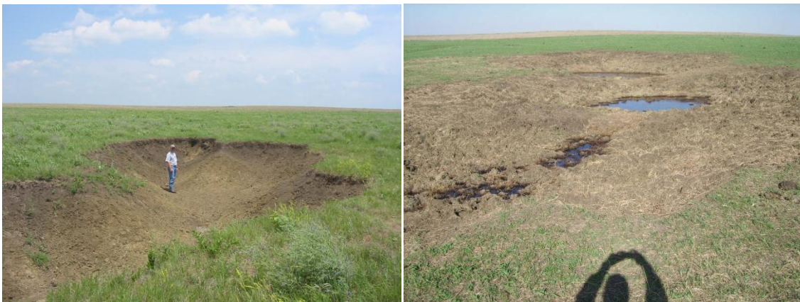
Dry Creek South Headcut, before (left) and after restoration construction.
